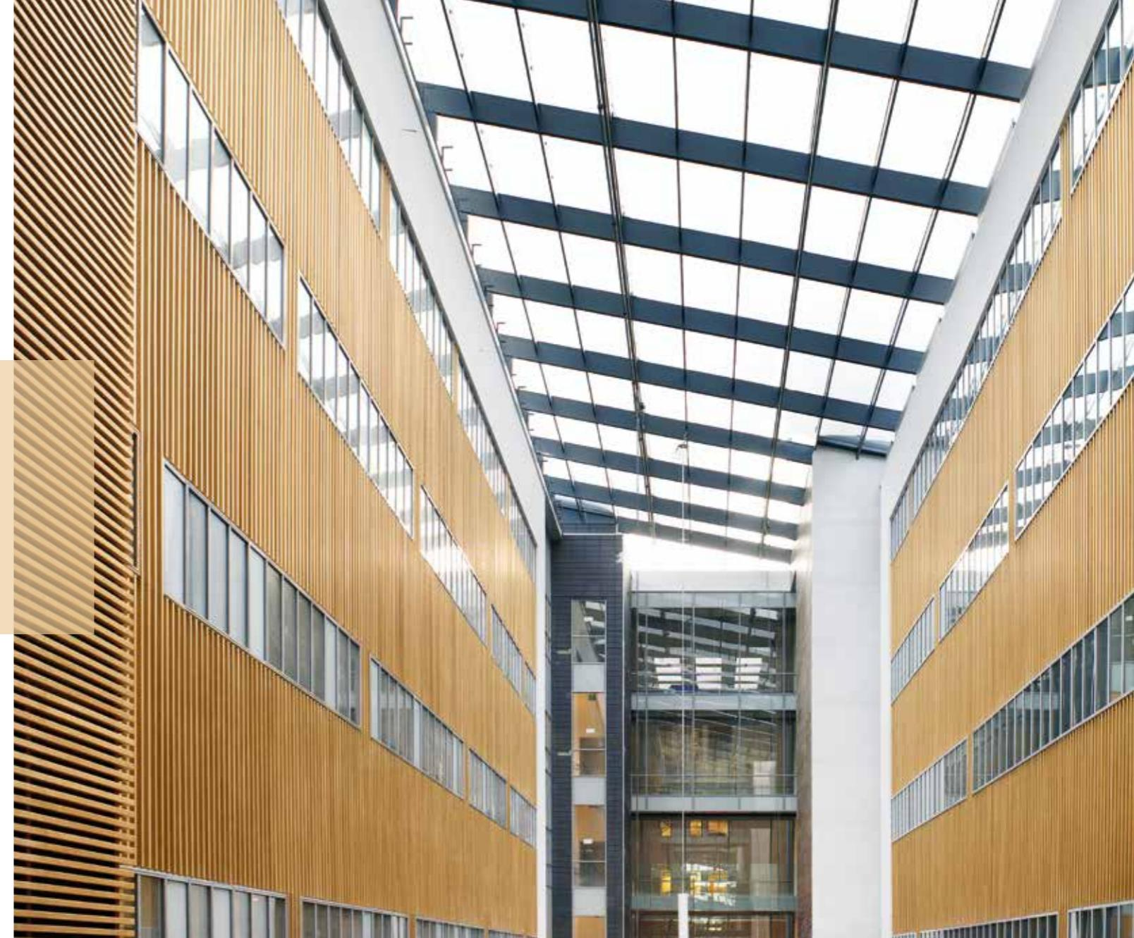
**FOR THE WALL APPLICATION A SPECIAL U-PROFILE IS USED.** The U-profile is attached to the surface - maximum 600 mm c/c - and the rib, with corresponding grooves, is then pressed onto the U-profile. A dab of carpenters glue is recommended in the grooves at installation. Final adjustment is done with a rubber mallet.
