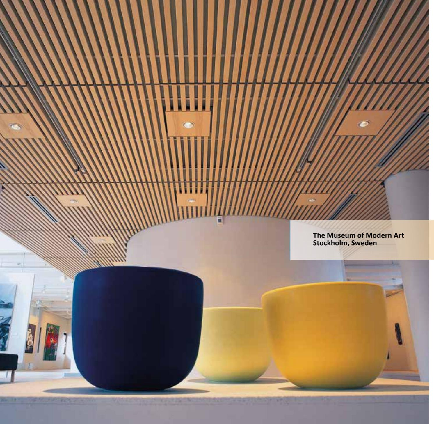
**DALHEM RIBBA IS A FLEXIBLE CEILING SYSTEM** for creative interior designs. The ribs have a substrate in particle gypsum board or MDF and are wrapped with real wooden veneer of the best quality.
